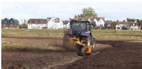
Image 5: Work begins at Conyer, where the restoration of coastal grazing saltmarsh is underway.
